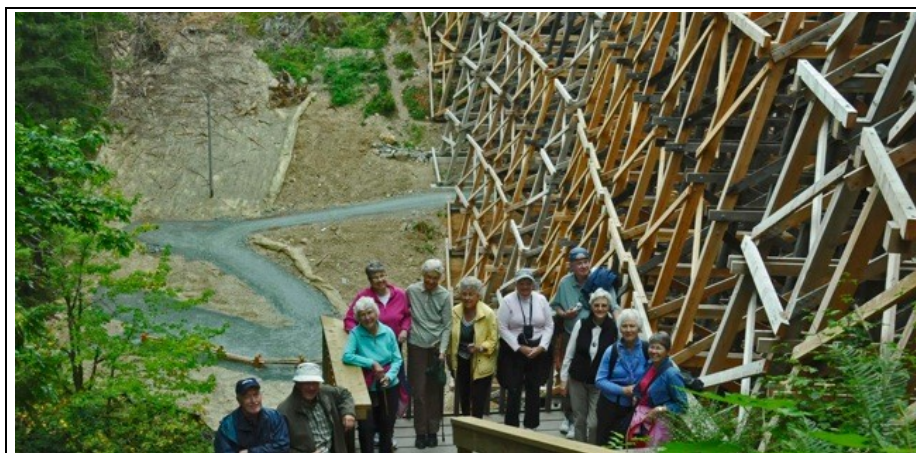
At the Kinsol trestle
